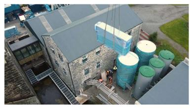
The combination of solar energy, hydro and very high temperature heat pumps, will make Ahascragh the first zero emission distillery in Ireland. Renewable heat and power specialists Astatine have developed and installed a revolutionary new system which will become the first in Ireland to use a heat pump above 100°C in Ireland, using water up to 120°C.
